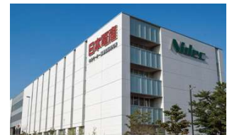
Nidec Research and Development Center, Japan Operates Entirely on Renewable Energies
