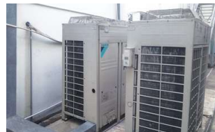
Nidec Tosok (Vietnam) Co., Ltd.'s air conditioning equipment with an energy-saving operation control system
