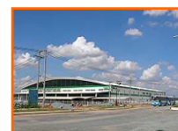
Production expansion at Nidec Vietnam
