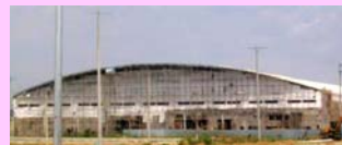
Nidec Vietnam under construction (Start-up in Jun. 06')
