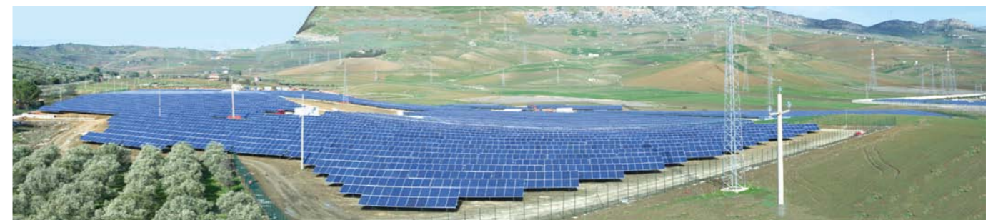
Photovoltaic power generation plant in a suburb of Cimenna, Sicily, Italy
