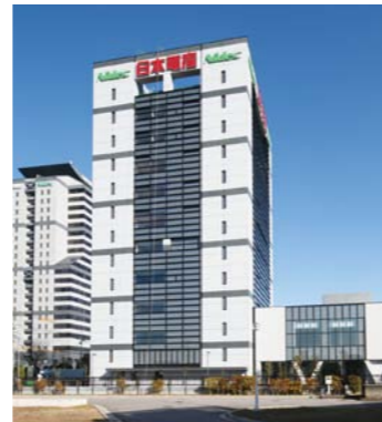
Nidec Corporation Head Office Annex Global Learning Center
